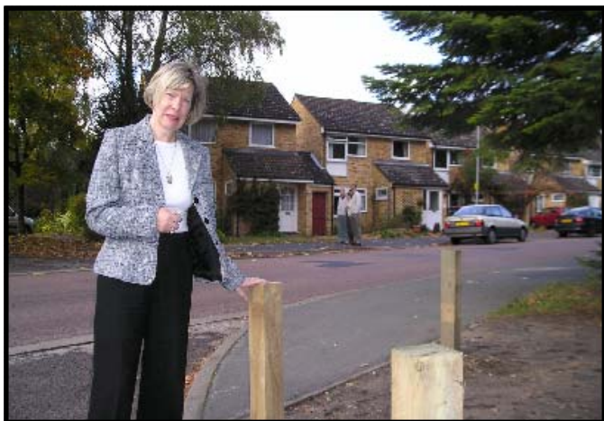
Fran inspects the installation of wooden posts to protect grass areas on Inglewood Avenue
